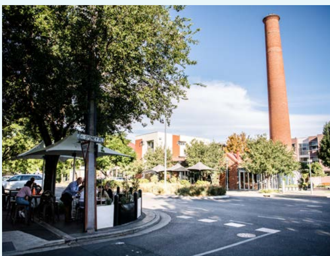
Former City Destructor Complex Heritage Adaption
