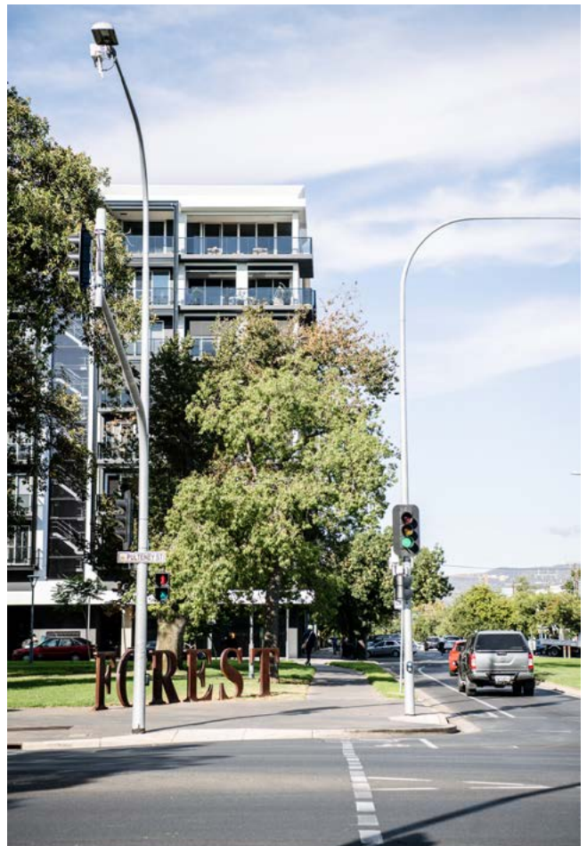
Recent development along South Terrace
